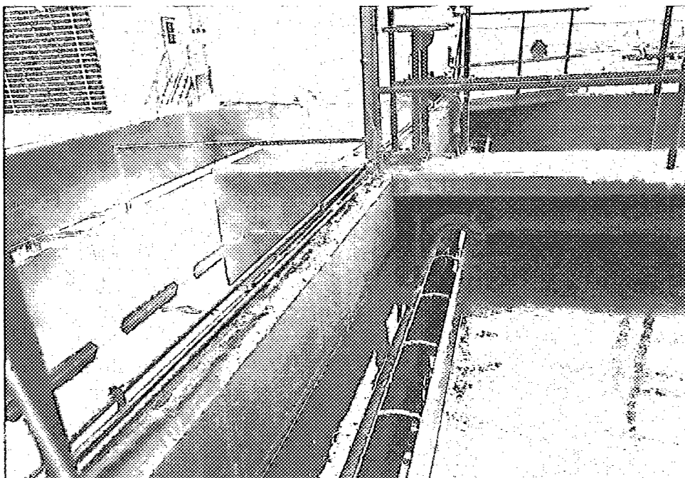
Figure 10—General Arrangement of Rotatable Slotted-Pipe Skimmer
