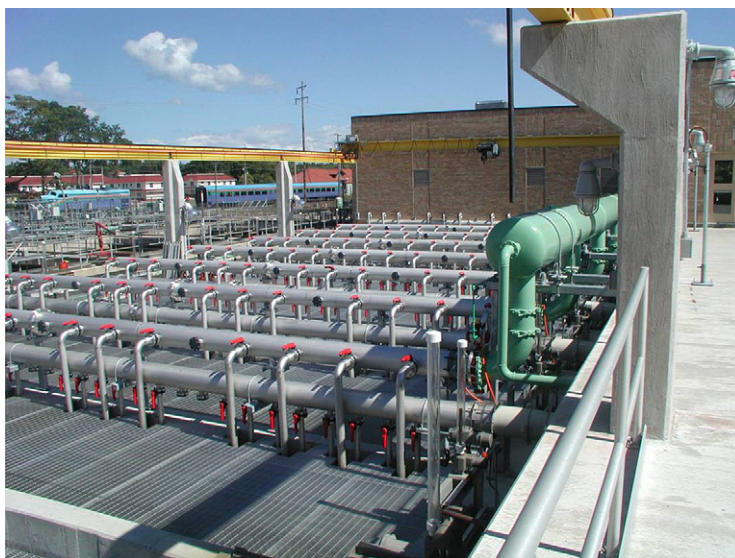
FIG. 5.35 The MBR at Traverse City WwTW, showing the permeate and air headers.
