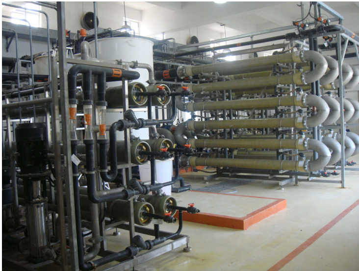
FIG. 5.55 The membrane skids at Baishi Ao, Foshan City: NF (left) and UF (right).
