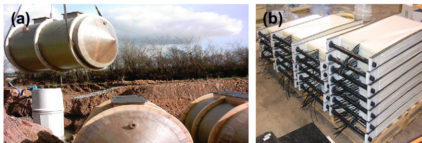
FIG. 5.16 (a) Installation of the tanks at Feenagh and (b) the membrane modules.
