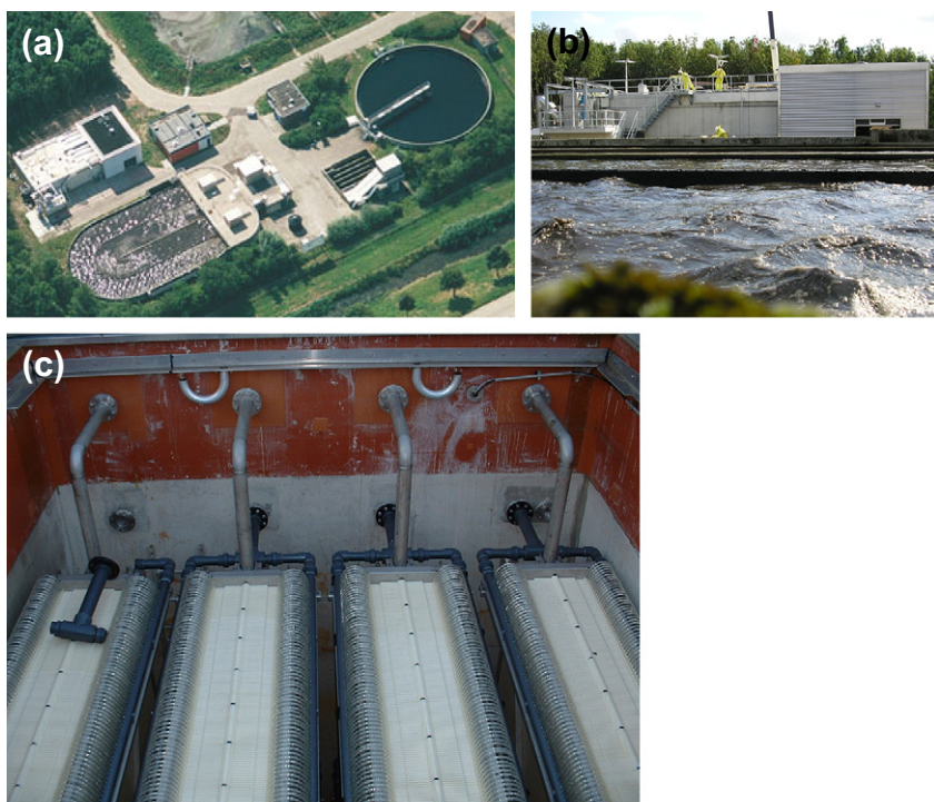
FIG. 5.21 Heenvliet WwTW: (a) from the air, (b) from the side and (c) inside the membrane tanks.
