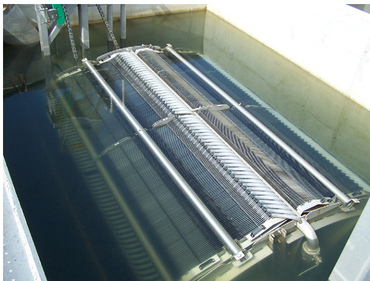
FIG. 5.18 The Huber VRM unit being installed at Arenas de Iguña.
