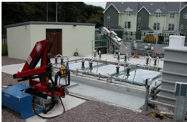
FIG. 5.15 The plant at Halfway. The screen is located mid/top picture, with the inlet pump chamber behind it. The anoxic tank is below the screen, and the MBR is the covered tank with the swan-neck air feed lines. The sludge tank is located behind the MBR and to the right of the anoxic tank. The permeate pump chamber is behind the sludge tank.
