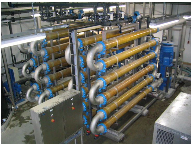
FIG. 5.51 The sidestream MT modules at Eemshaven.
