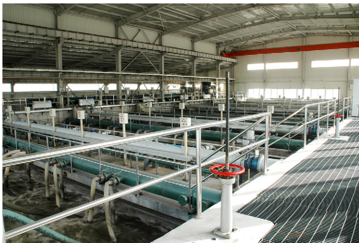
FIG. 5.49 The membrane tanks at Miyun.
