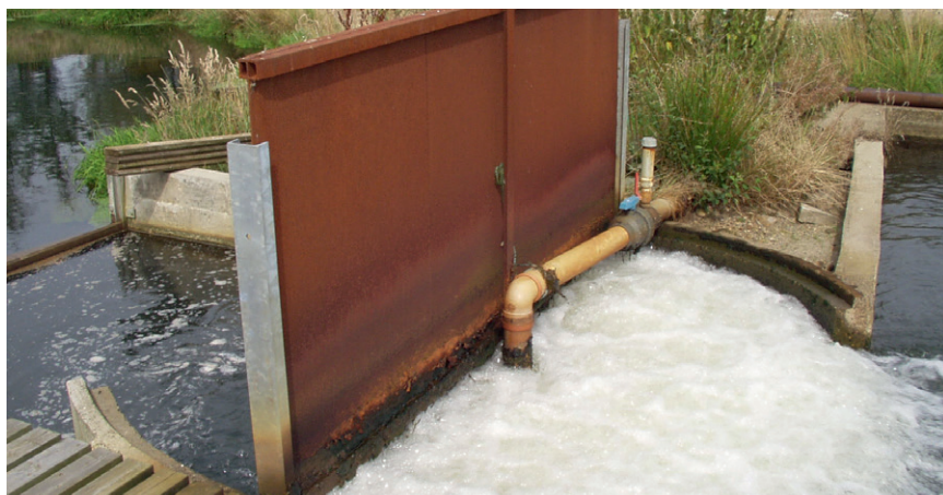
Figure 2.12 Aeration well system.
