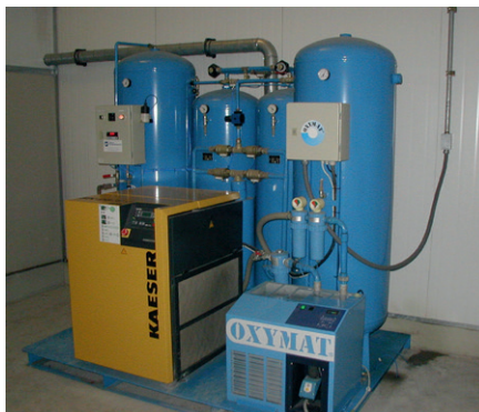
Figure 5.2 Oxygen generator. Control and service of special installations must be taken care of.
