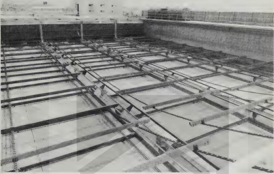
FIGURE 9-17 Empty rectangular sedimentation tank showing sludge removal flights.
