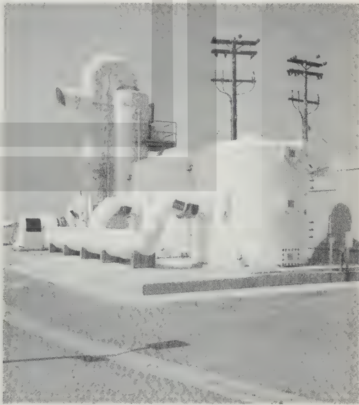
FIGURE 9-36 Typical activated-carbon system for odor control: (a) schematic and (b) typical installation.
