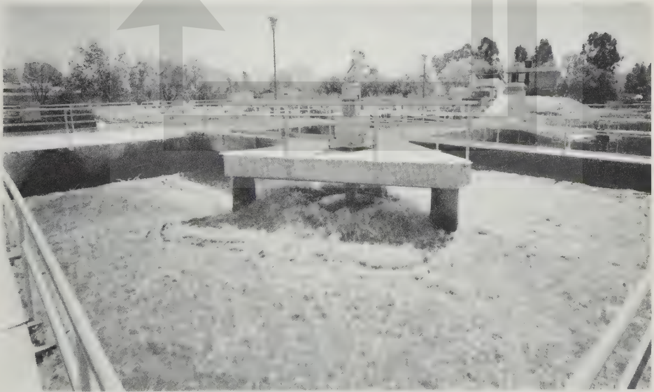
FIGURE 8-14 Typical complete-mix activated sludge reactor with surface aeration.
