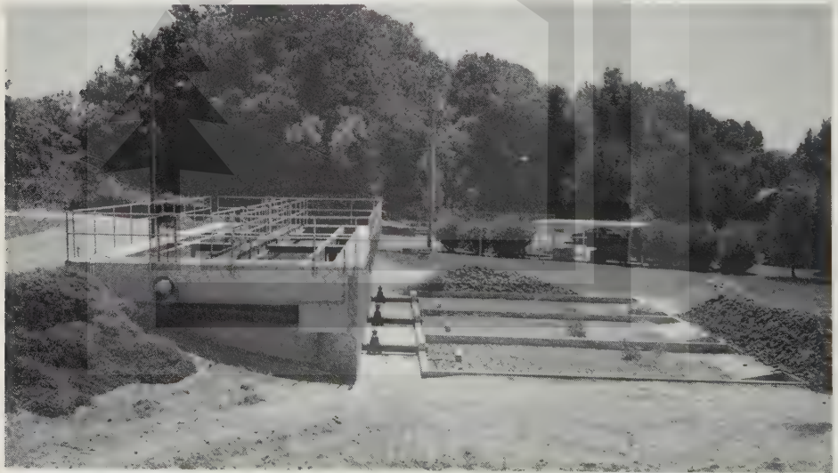
FIGURE 14-27 Typical Imhoff tank used for a small community. Effluent from the Imhoff tank is disposed of in a series of rapid infiltration basins. Note sludge drying beds located adjacent to the Imhoff tank.
