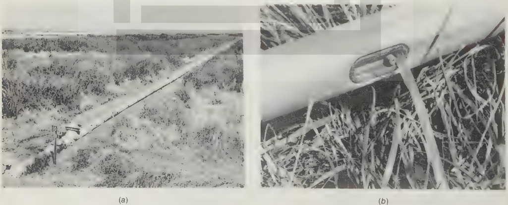
FIGURE 13-11 Gated aluminum pipe used for wastewater distribution: (a) typical installation and (b) close-up of adjustable discharge port.
