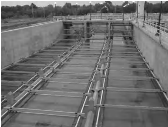
Figure 10-12 Chain-and-flight-type sludge collector.
