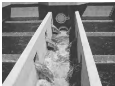
Figure 11-1 Typical dual-media rapid filter. (a) Schematic representation of dual-media filter. (b) View of an operating rapid filter. Washwater troughs are visible below the water surface. Influent water enters through the central channel, flows through the wall openings for the washwater troughs, and then down through the filter media, which is below the water surface. (c) Rapid filter during the backwash cycle. Washwater flows up through the media, pours over into the troughs, and then runs into the central channel.
