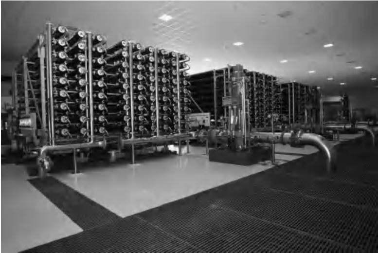
Figure 17-2 Typical reverse osmosis facility.
