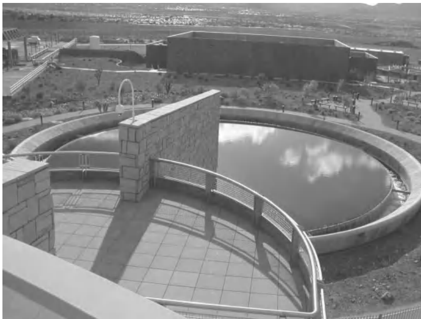
Figure 23-13 Flow-splitting basin, viewed from above.
