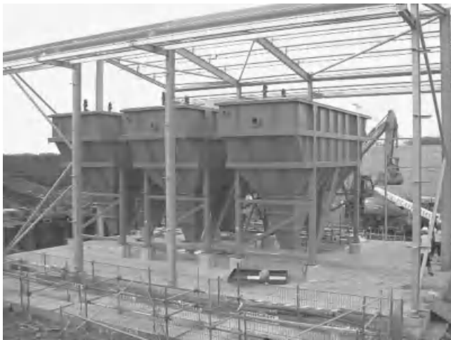
Figure 23-10 Lamella-plate settling modules provide washwater treatment prior to recycle.
