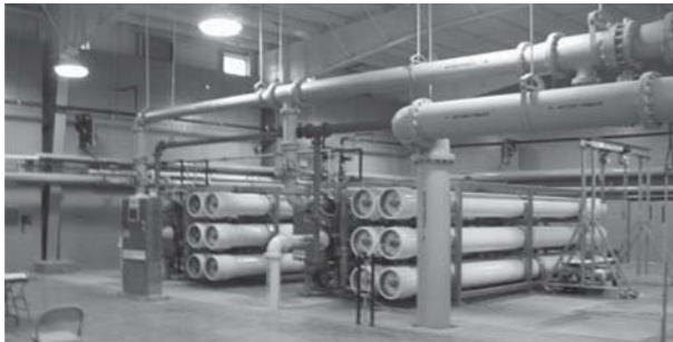
Figure 4.25 Two-train MegaMagnum RO system. Each train is capable of providing 1,390 gpm product flow when a 28-mil spacer is used, and 1,340 gpm when a 31-mil spacer is used. Courtesy of Koch Membrane Systems.
