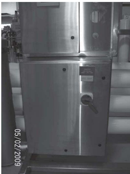
Figure 6.5 Variable frequency drive (VFD) control cabinet. Courtesy of Nalco-Crossbow Water LLC.
