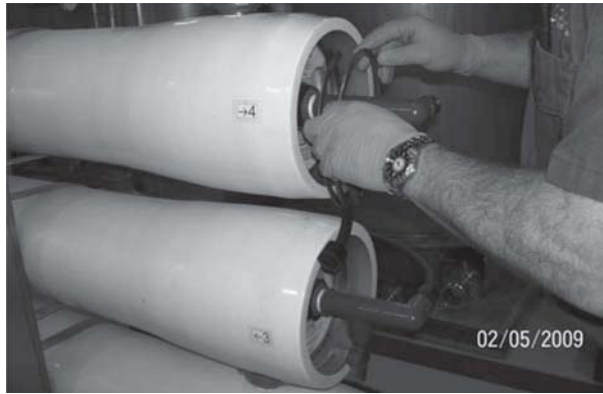
Figure 6.14 Snap ring that holds pressure vessel end cap in place. Courtesy of Nalco-Crossbow Water LLC.
