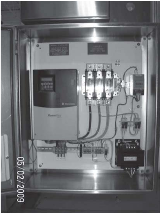
Figure 6.6 Inside of a variable frequency drive (VFD) control cabinet. Courtesy of Nalco-Crossbow Water LLC.
