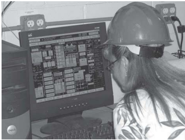
Figure 6.17 Human-Machine Interface (HMI) showing status of the reverse osmosis system, including pretreatment.
