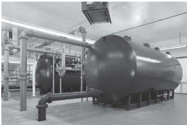
Figure 8.8 Horizontal multimedia pressure filter with 4 internal cells. Courtesy of Siemens Water Technologies Corp.
